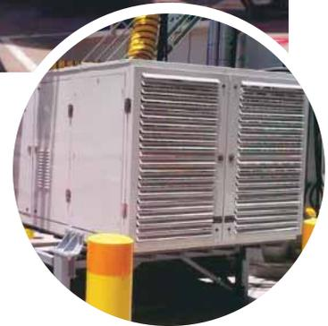
AOT installed Fixed Ground Power Units and Fixed Pre-Conditioned Air units (PC AIR) for 51 parking bays at Suvarnabhumi Airport to provide power supply and cooling for aircraft. This technology enables AOT to reduce air polluting emission and extend the life of aircraft equipment by eliminating the need to keep engines running. AOT is planning to install additional units at all parking bays at Suvarnabhumi Airport and other airports in the future.
